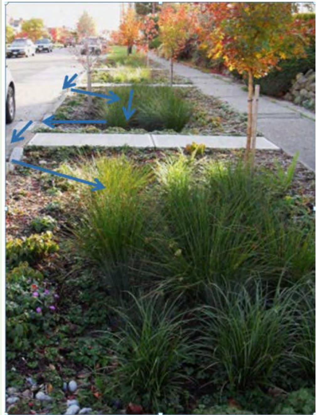
Figure 5. Typical Flow Pathway through the 30th Avenue Raingarden
