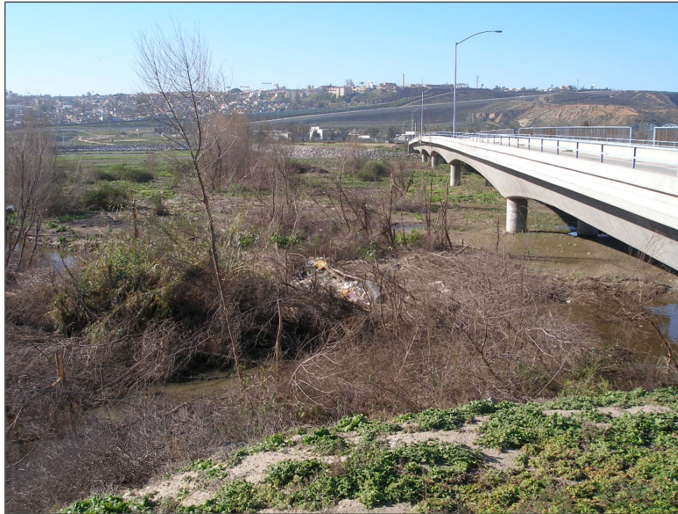
The forest at Dairy Mart Bridge after the beetle attack (February 2016).
